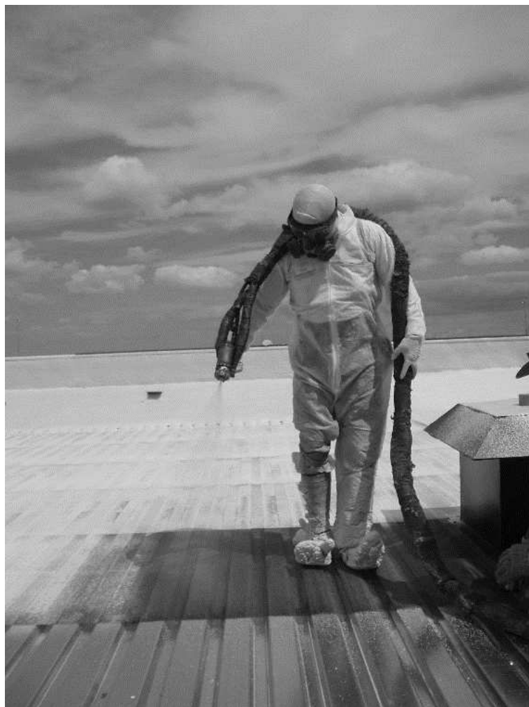
Spray Foam Roofing application.
