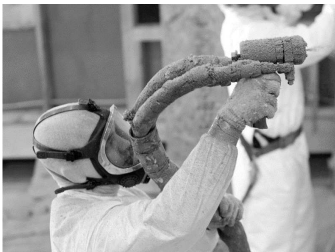
Spray Polyurethane Foam installation
